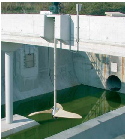
WEEDLESS-V agitators consist of a geared motor above water level and a propeller positioned below.
