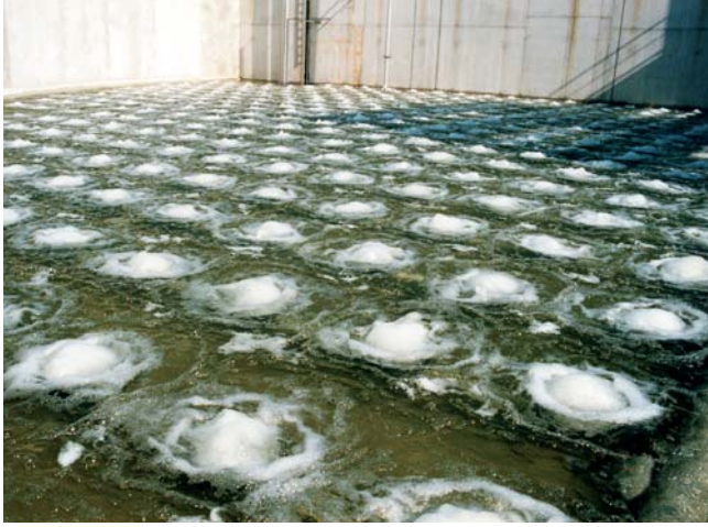
The membranes of ELASTOX®-T disk air diffusers consist of a special composition rubber (EPDM) or special silicone that have already proved their worth in many facilities.
