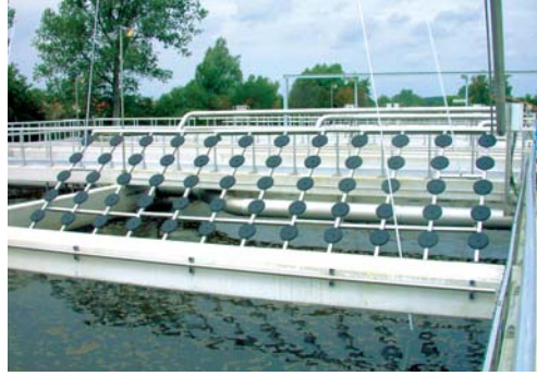
Removable aeration field with ELASTOX®-T disk air diffusers
