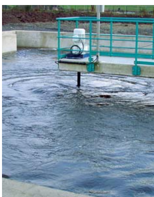
WEEDLESS-V vertical agitators are simply suspended from above in the tank.
