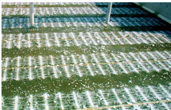
The low-buoyancy ELASTOX®-R tube air diffuser design is based on the floodable support tube principle.
