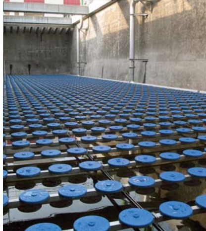
ELASTOX®-T disc air diffuser membranes are manufactured from special rubber (EPDM) or special silicone that has proven its effectiveness in a multitude of systems.
