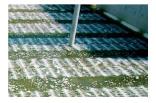
A great many oxygen admission tests on existing facilities have confirmed that ELASTOX<sup>®</sup>-R tube air diffuser take a leading position as to micro-bubble aeration systems.
