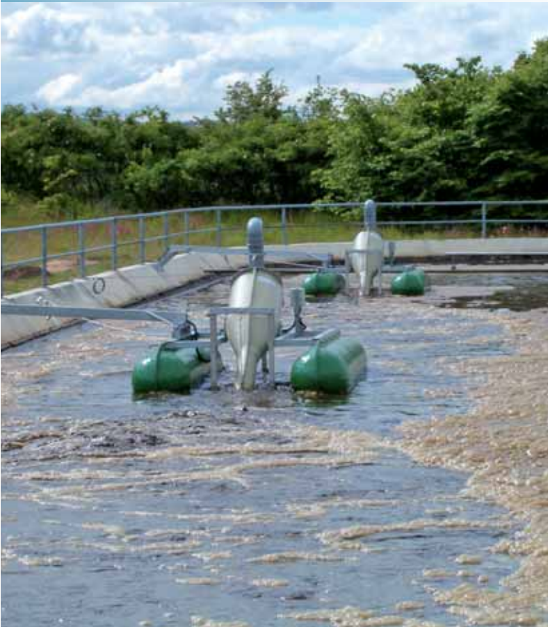
FUCHS Aerators on floats adapted to an oxidation ditch
