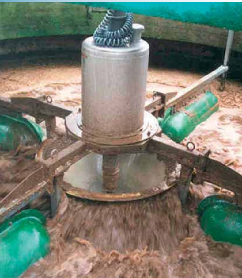
Retrofit for sludge stabilization in a converted storage tank
