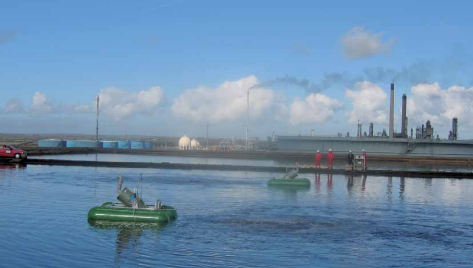
Treatment of petro-chemical effluent in a large lagoon system
