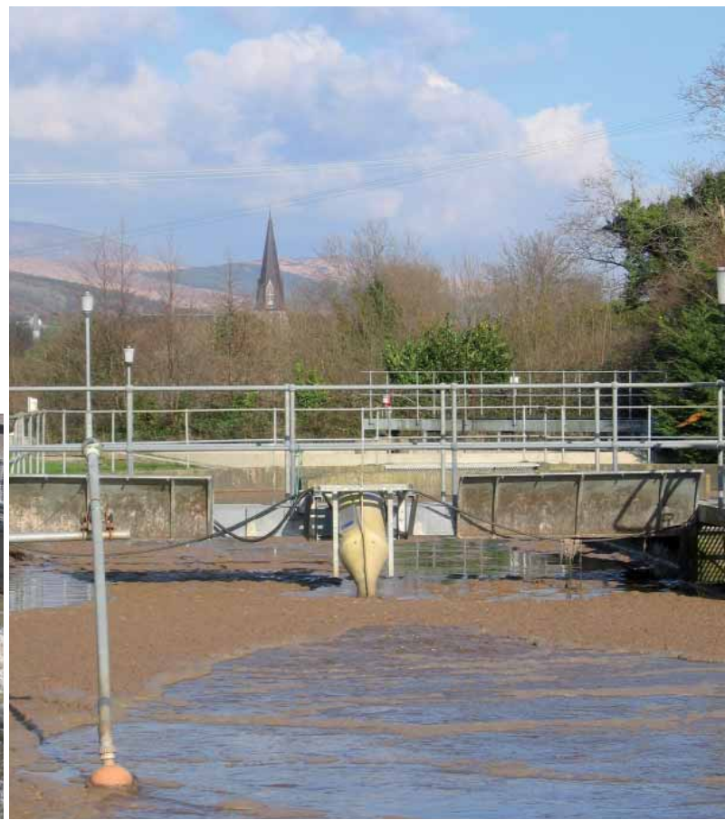
Replacement of old high-maintenance rotors with a FUCHS Spiral Aerator
