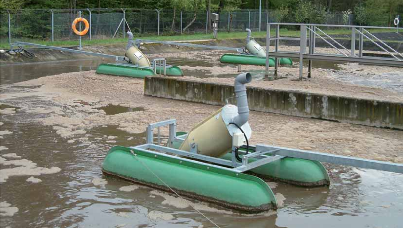
FUCHS Aspirating Aerators on floats meet the oxygen deficit of an inadequate aeration system
