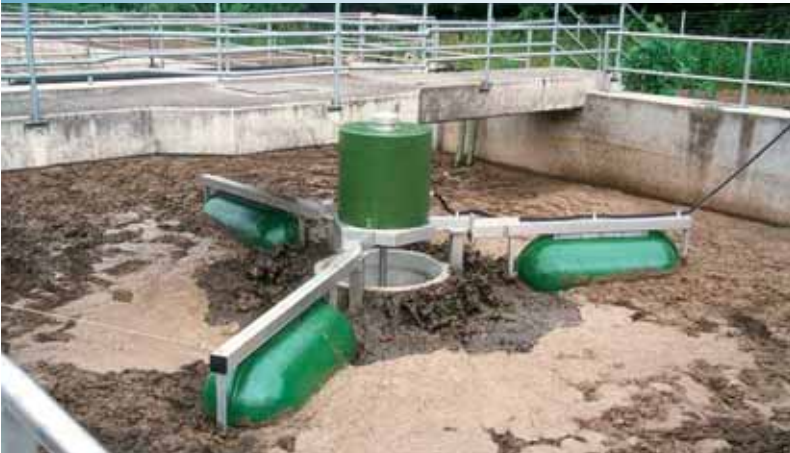
Aerobic stabilization of sewage sludge in a former storm water tank
