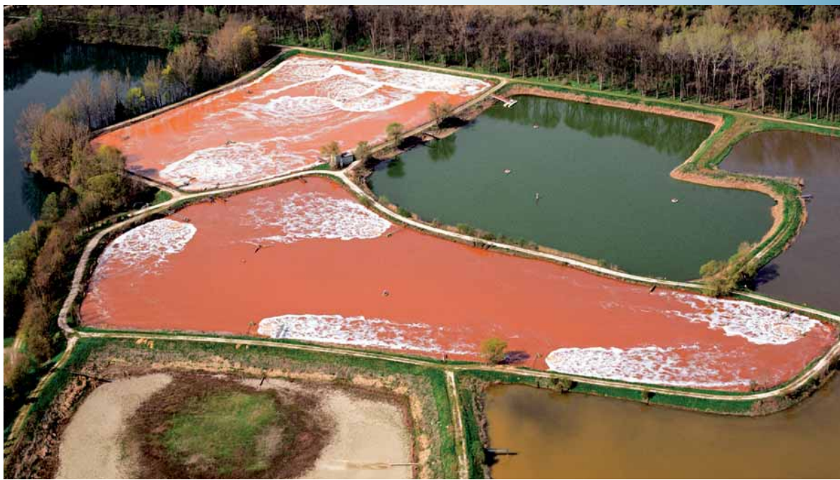
Strongly directional flow pattern created in sugar mill lagoons by FUCHS Aspirating Aerators
