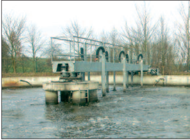
OLD: COUNTER CURRENT AERATION SYSTEM
