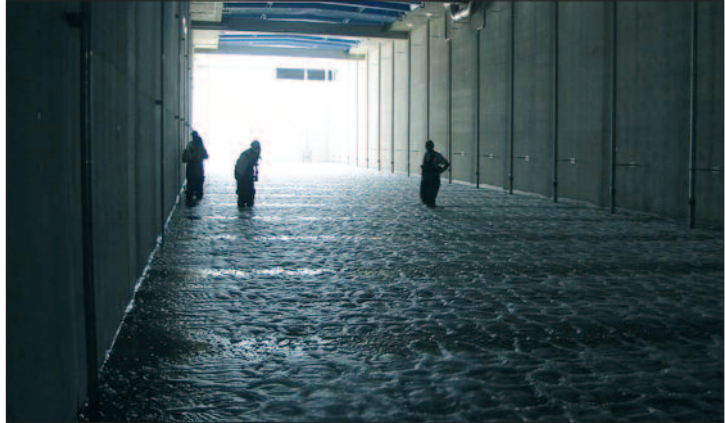
OTT MEMBRANE TUBE DIFFUSERS AT HOECHST INDUSTRIAL PARK, FRANKFURT AM MAIN
