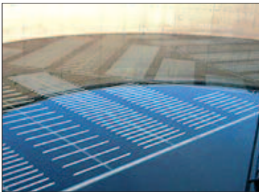
NEW: FULL FLOOR COVERING, EFFICIENT OTT HE® AERATION
