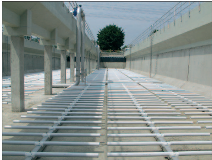
HANAU WASTEWATER TREATMENT PLANT: AERATED WITH OTT MAGNUM® FLEXSIL® HE® MEMBRANE DIFFUSERS
